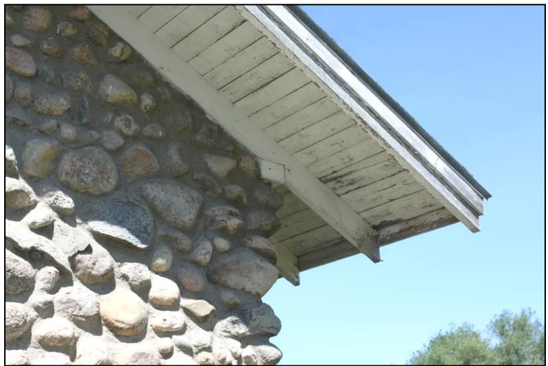
Detail showing stonework and soffit.
