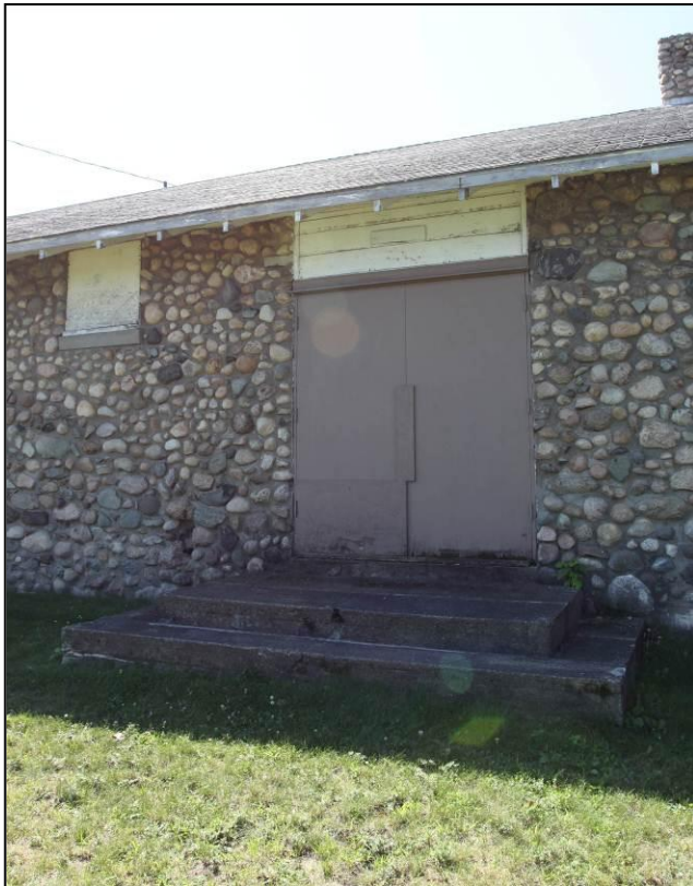
Below: View of main entrance on north facade showing double-door entrance with transom and concrete stair. View to southeast.
