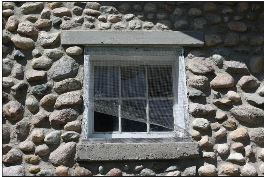
Detail view of window opening showing six-light hopper window, concrete sill and lintel, and attached screen material.
